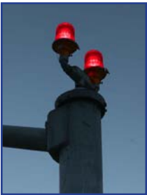
[Left] Red boundary beacons for Torrance Airport in California, mounted atop perimeter luminaire poles; [Below] Blue accent lighting atop poles on Chicago's State Street
